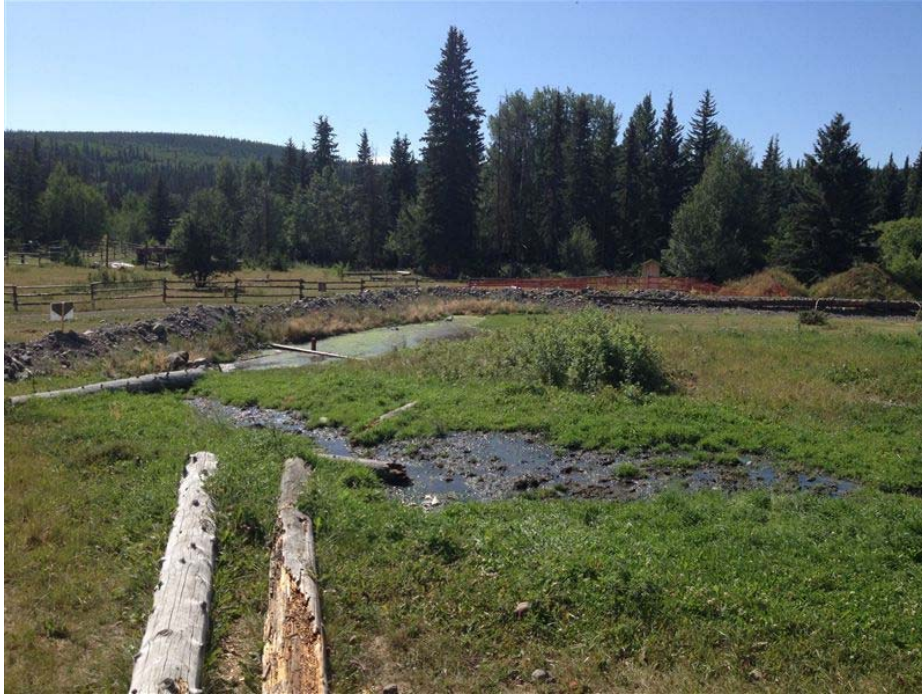
The community's failing septic field.
