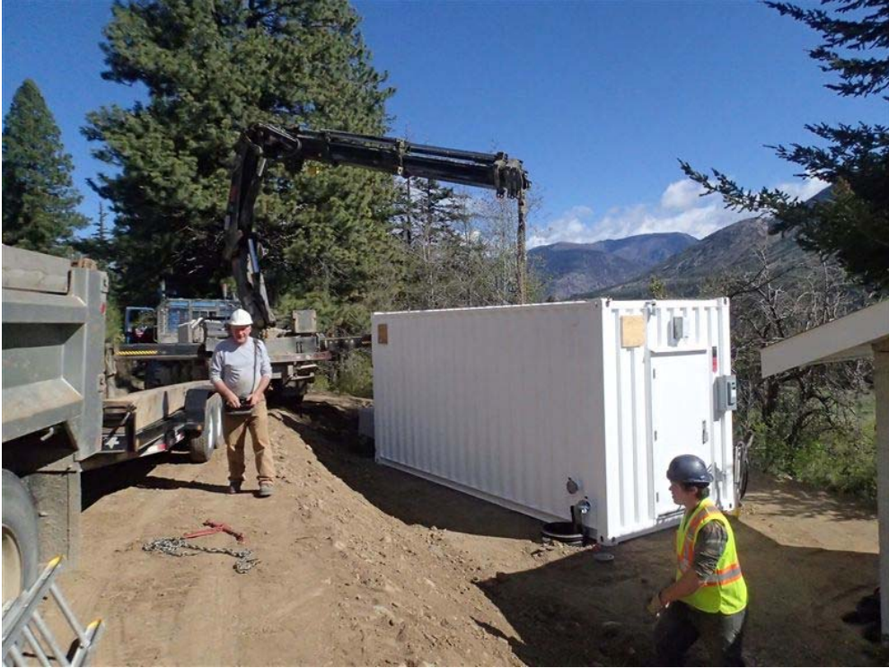
The new plant is lowered into place.
