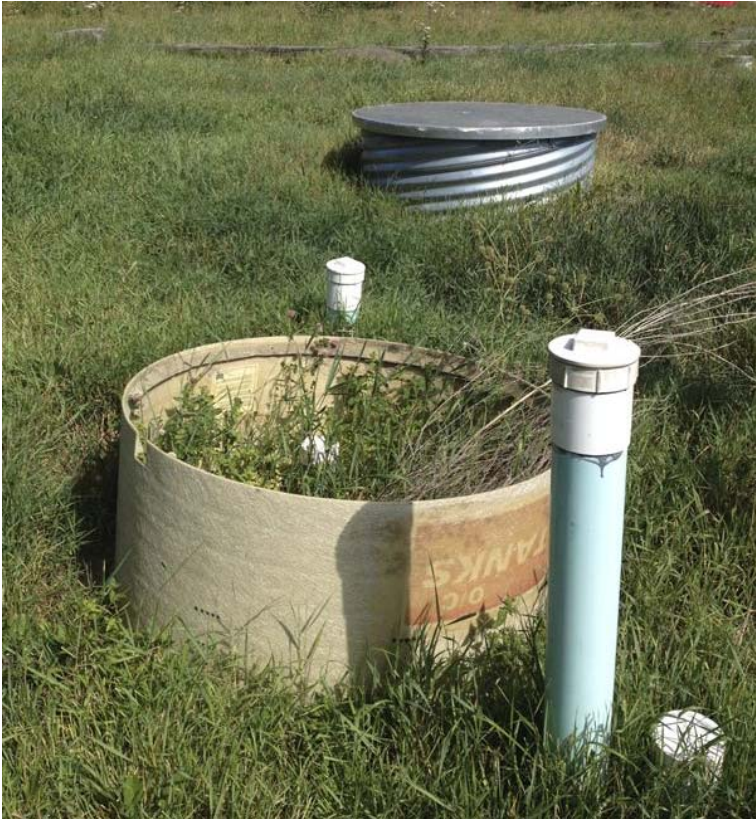
The former septic system.
